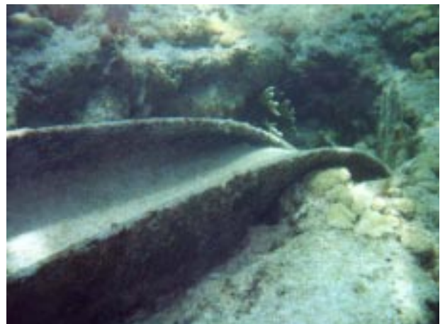
Hurricane Georges bent and broke some stout I-beams that once support the Looe Key marker
