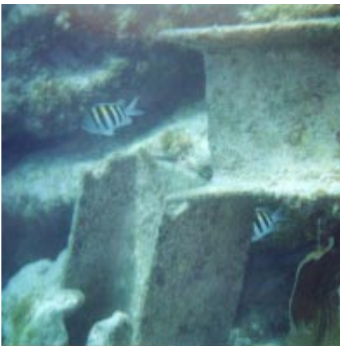
Hurricane Georges bent and broke some stout I-beams that once support the Looe Key marker
